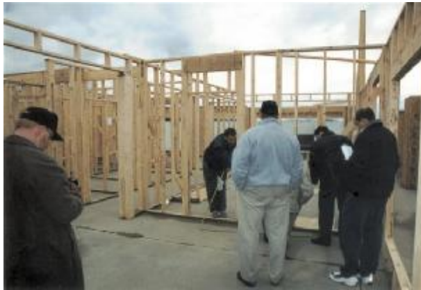
Figure 1 An example of a physical mock-up (PMU) used for a design review session (courtesy of Pulte Homes, Inc.)
