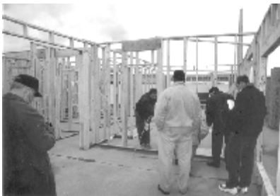
Figure 2: An example of a physical mock-up used for a design review session (Courtesy of Pulte Homes, Inc.)
