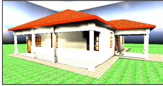
Fig. 8 Rear view of the prototype house.
