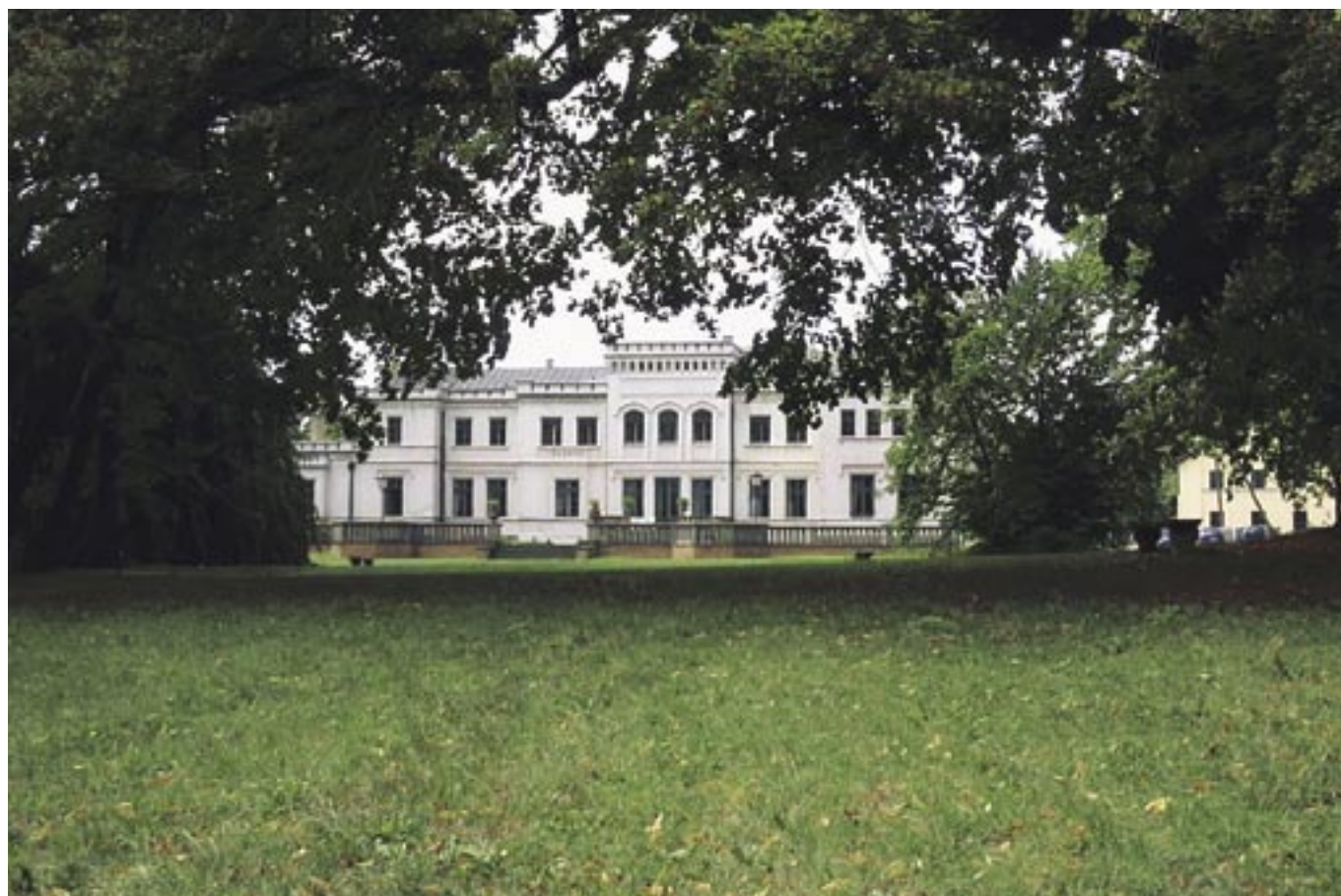
The palace containing dining rooms.
