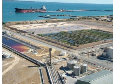
Figure 4: An aerial view of the treatment train at CSBP. Alternate fill-and-drain operation is visible on the two VF parallel cells (far end) just prior to planting. Note the transverse vegetation strips on the saturated VF wetland as a result of removal of the top sludge layer to overcome clogging.
