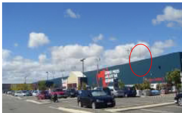
Figure1. A photograph of the front view of the Bunnings warehouse showing the five small wind turbines and the ultrasonic anemometer position (red circle)
