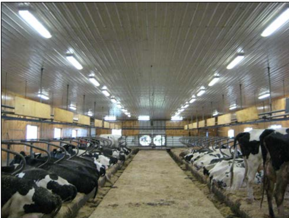
Fig.7. New section of the primary facility with T8 fluorescent lighting.
