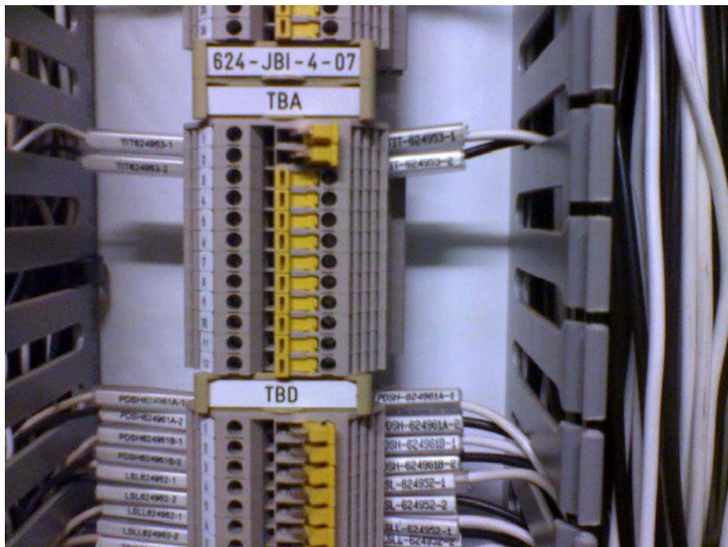
Figure 5: Physically ferruled cables
