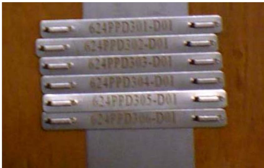
Figure 8: Cable Tags for Multipair Cables
